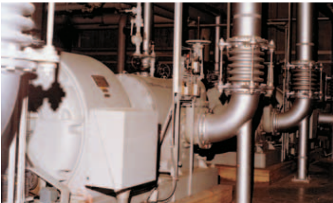
Two (2) model 23D Ro-Flo® vacuum compressors recovering propylene oxide for a confidential user in Italy. 2513 acfm of gas is being compressed from 8.9 psia to 36.7 psia using a 250-hp motor at 495 rpm.
